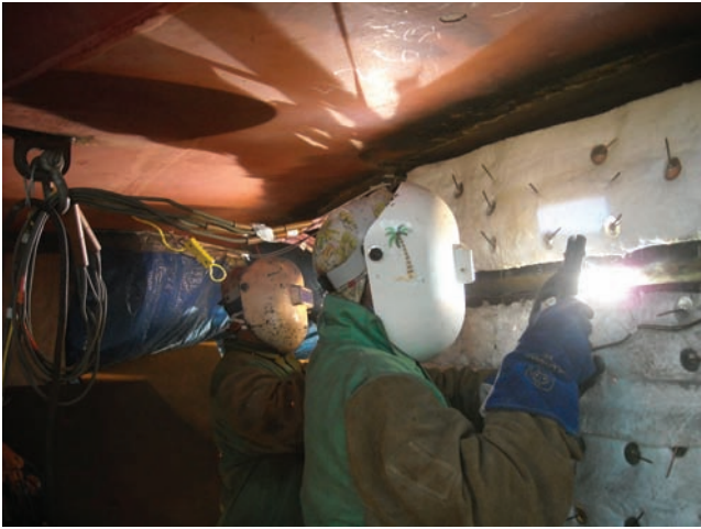
Fig. 10 — Two welders working simultaneously on the portside joint.
