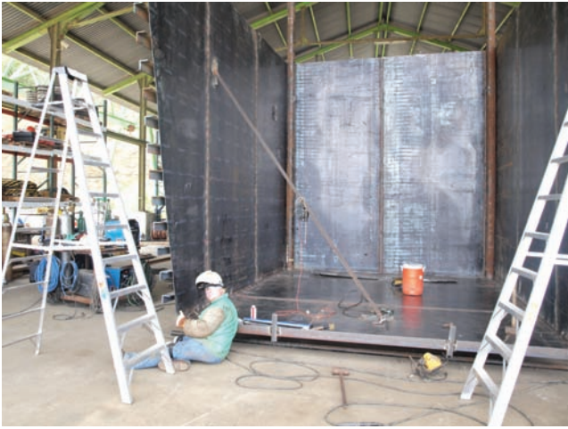
Fig. 6 — Welder Bruce Smythe at work building the 23,000-lb cofferdam.
