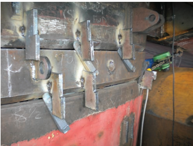
Fig. 8 — Joint preparation on the insert on the port side.
