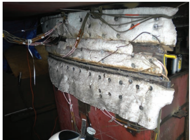
Fig. 9 — Ceramic heating elements and insulation are shown installed at the joint to be welded.
