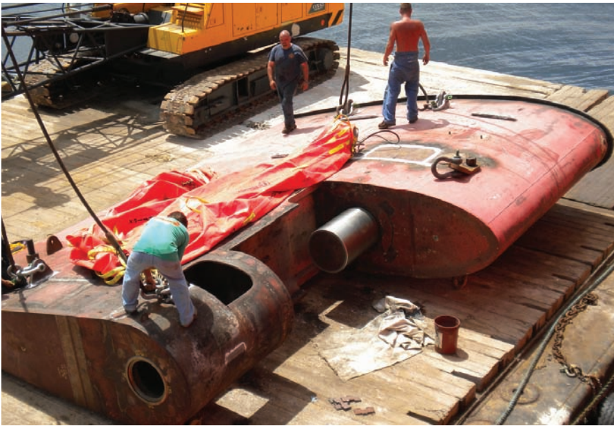
Fig. 12 — The rudder on the barge deck awaiting reinstallation.
