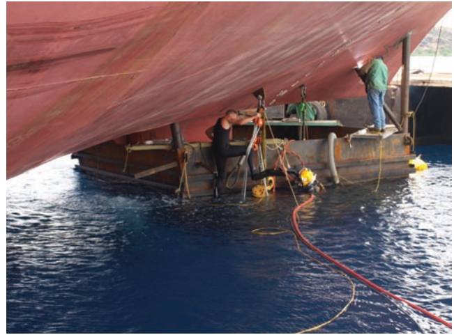
Fig. 7 — Installing the cofferdam.
