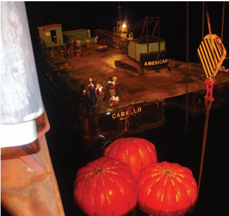
Fig. 3 — The rudder hanging from the lift bags.
